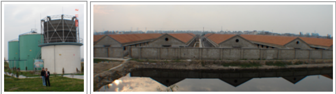
A Chinese 12,000 heads piggery with all manure converted to slurry and biogas © 2003, Pauli
