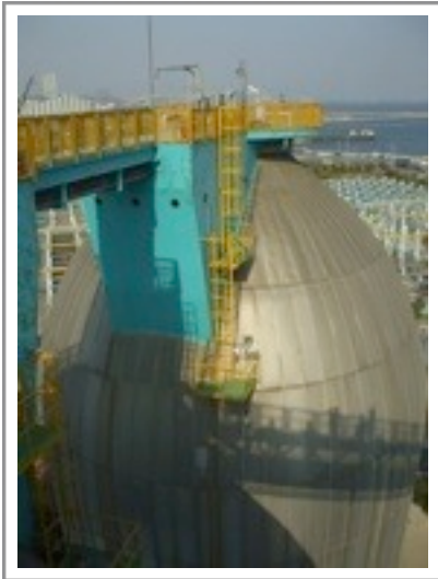
Digesters at the Ulsan waste water treatment plant designed by Scandinavian Biogas © 2011, Scandinavian Biogas
