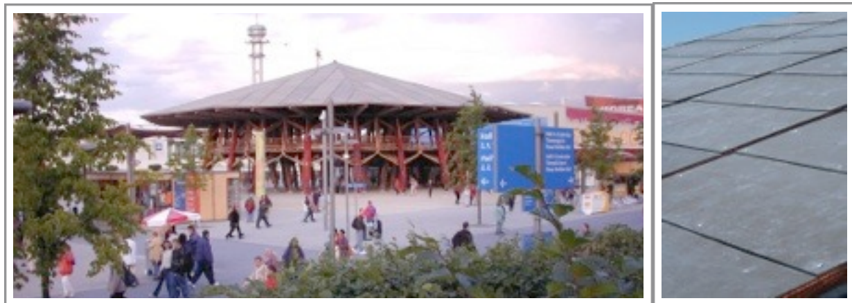
The ZERI Pavilion at the World Expo 2000 in Hanover with the first ever bamboo/cement fiberboard roofing © 2000, Pauli
